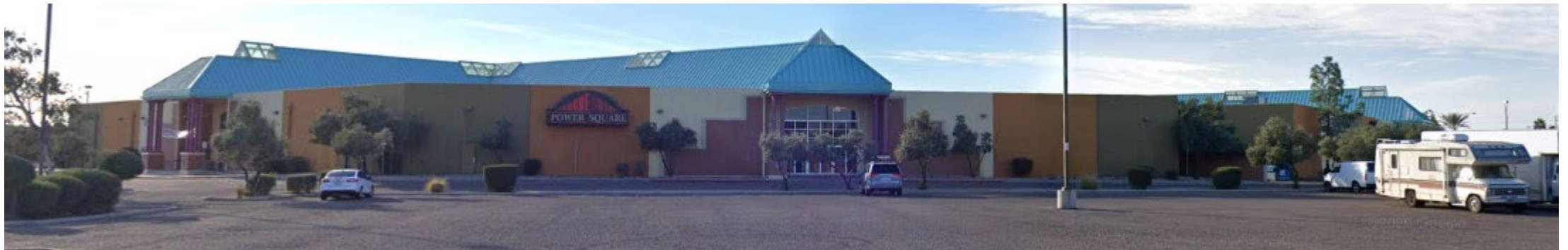
Looking east from Power Road
